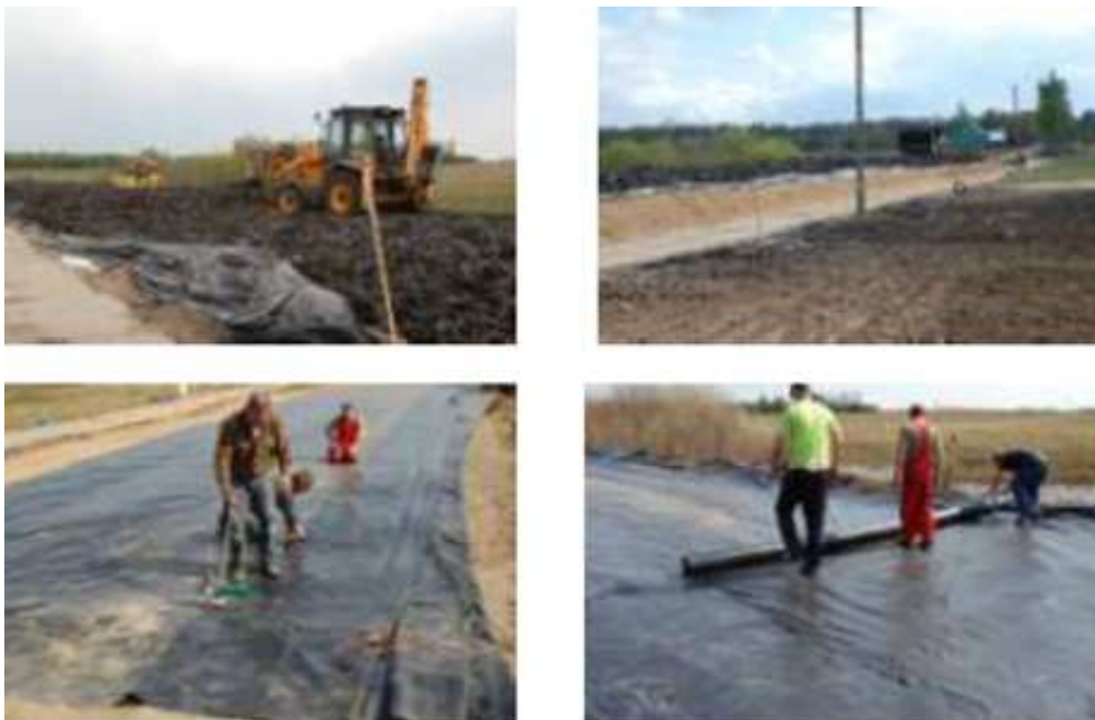
Figure 19: Construction process of Rectyre embankment in Czuprynowo
