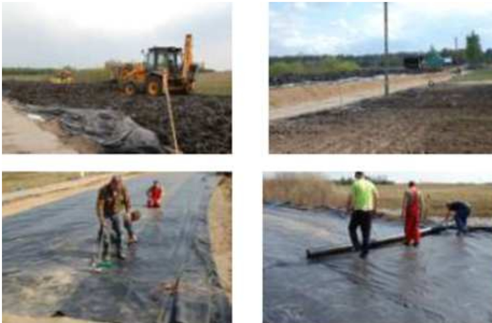
Figure 19: Construction process of Rectyre embankment in Czuprynowo
